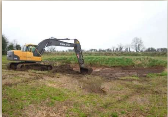
Pond being excavated in the Bride Valley
