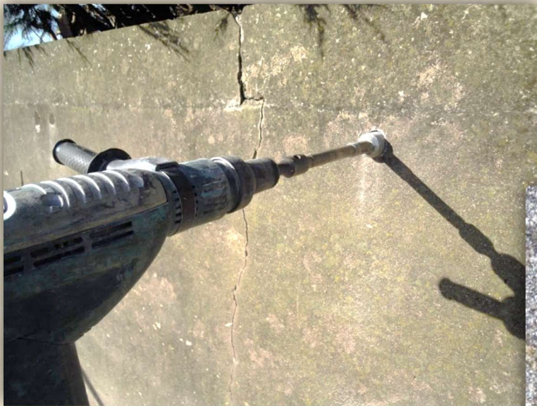
Drilling a hole in a cavity block wall can make a very effective nest box
