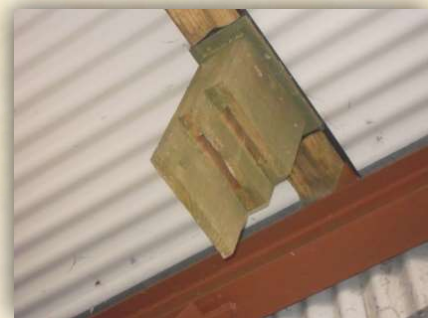
Bat Roosting Box
